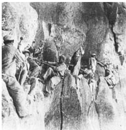
PLA soldiers building road by the Nujiang River
